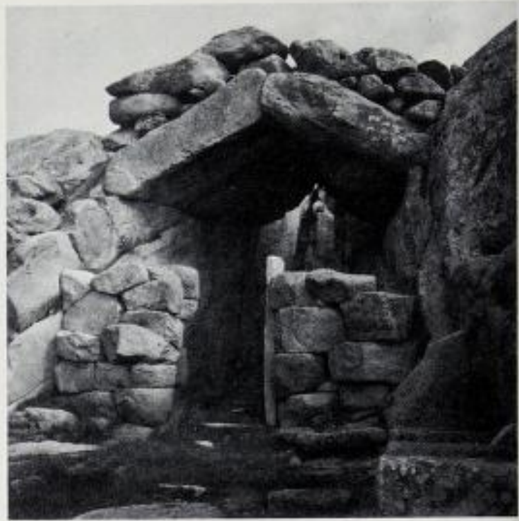
Arch construction in the Old World on the principle of the 'false arch'
